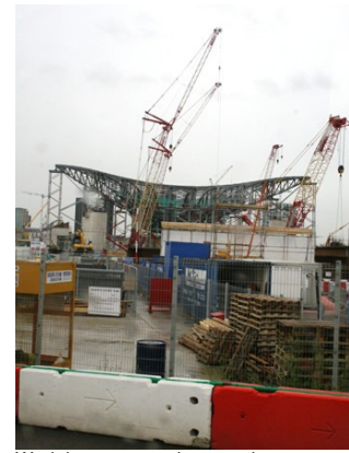
Work in progress: the aquatic centre
